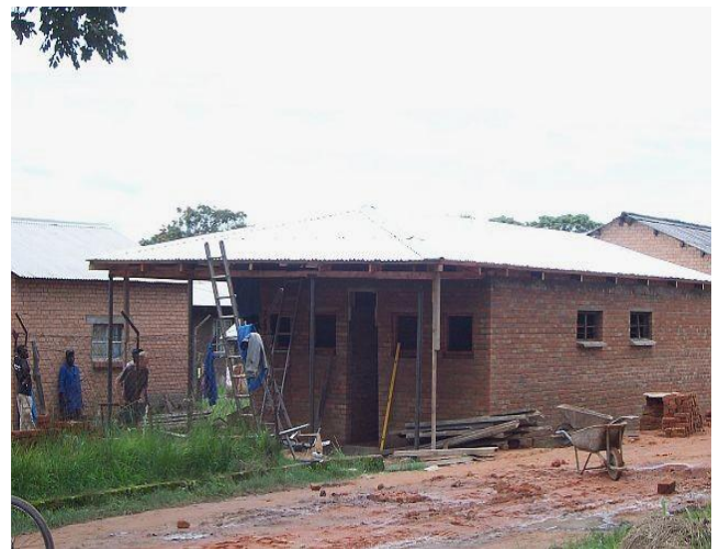
New CHAZ HIV block, with ablutions, offices and store room
