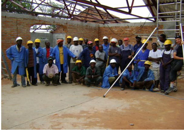
The Roofing team
