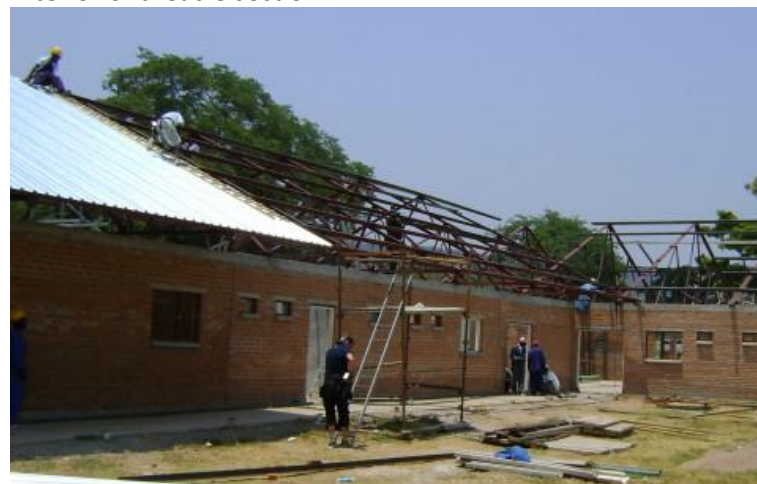
Placement of iron roofing sheets
