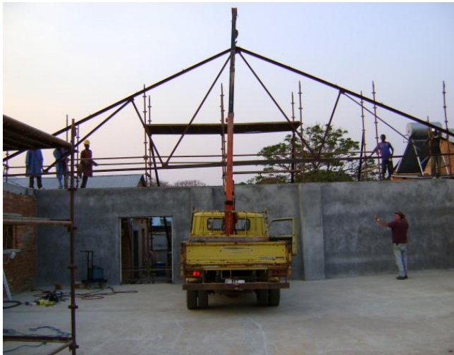
First truss being lifted into position
