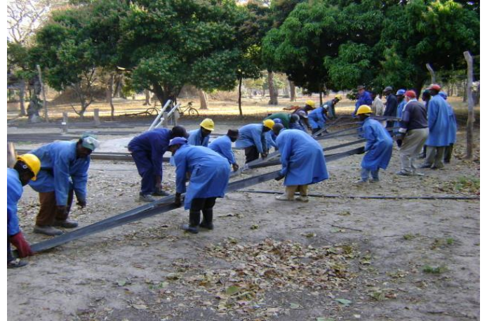
Lifting a welded roof truss for placement in new building
